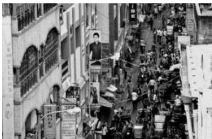
Illegal constructions in Sowcarpet/
